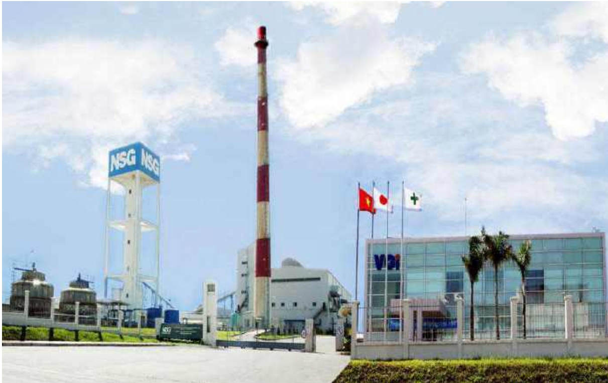
Upgrade the Gas safety system NSG Glass factory
