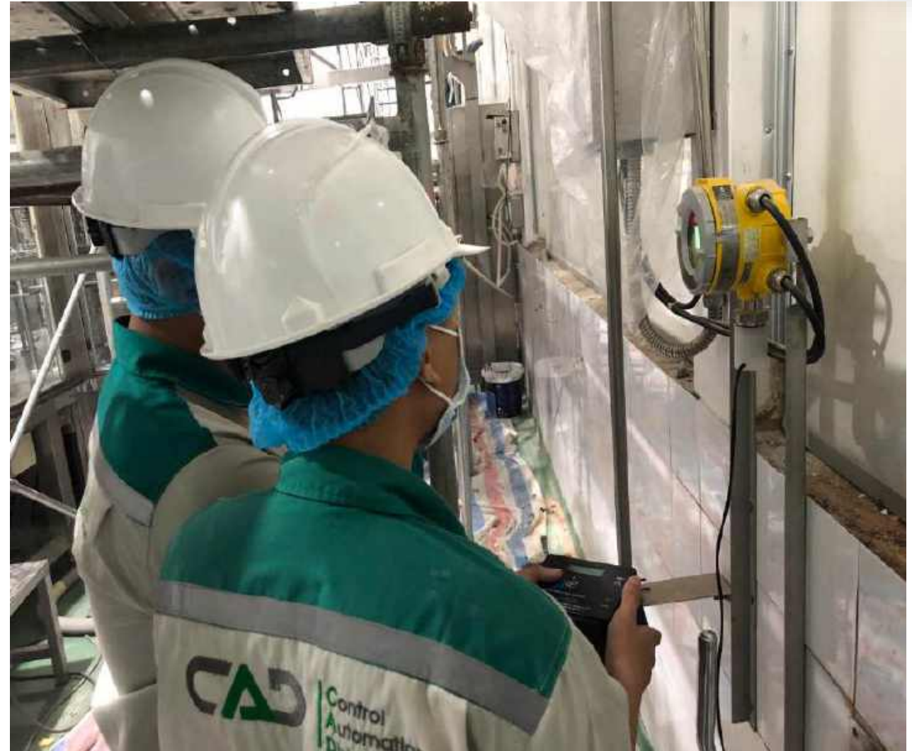
Upgrade the Gas safety system Nuplex Chemical factory
