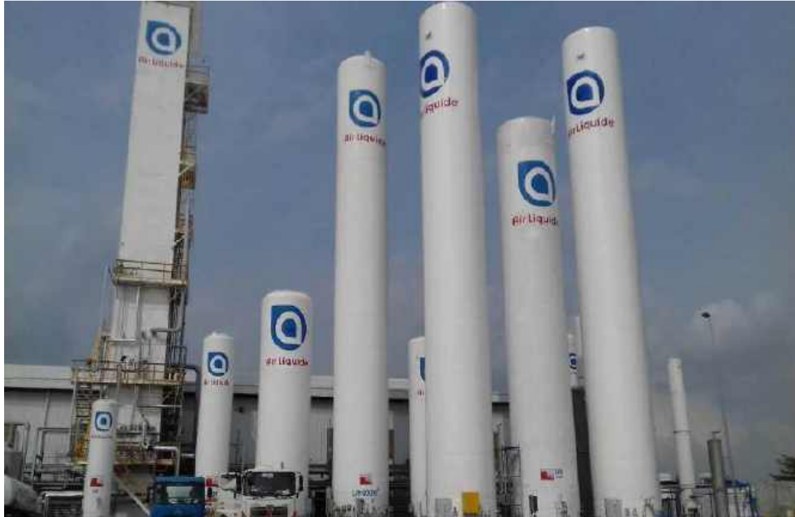
Upgrade the Gas safety system in Air-liquid factory
