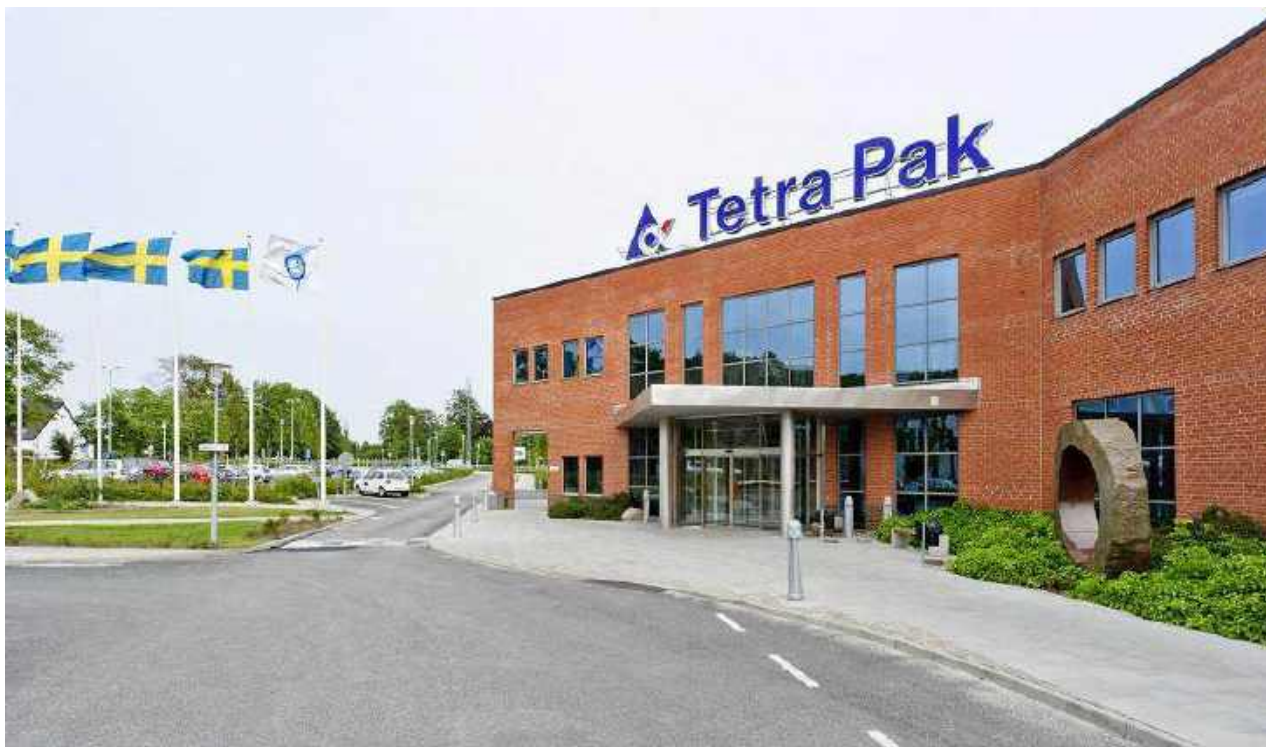
Upgrade the Gas safety system TETRA PAK factory
